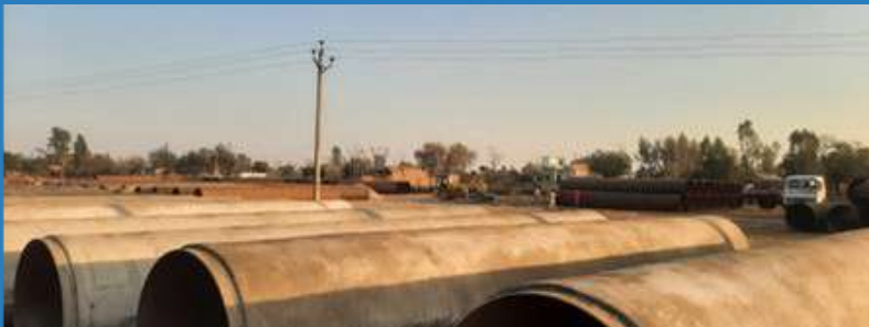
Guniting / Concrete Coating on irrigation pipeline – JayPee Associates – Rewa MP
