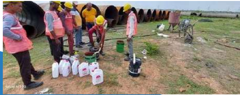
Irrigation Pipeline p rotective Coating at TATA Projects Lmt. MP
