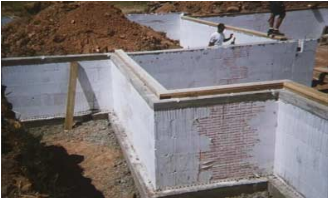
Corbels on the inside can be used for bearing joists, etc.
