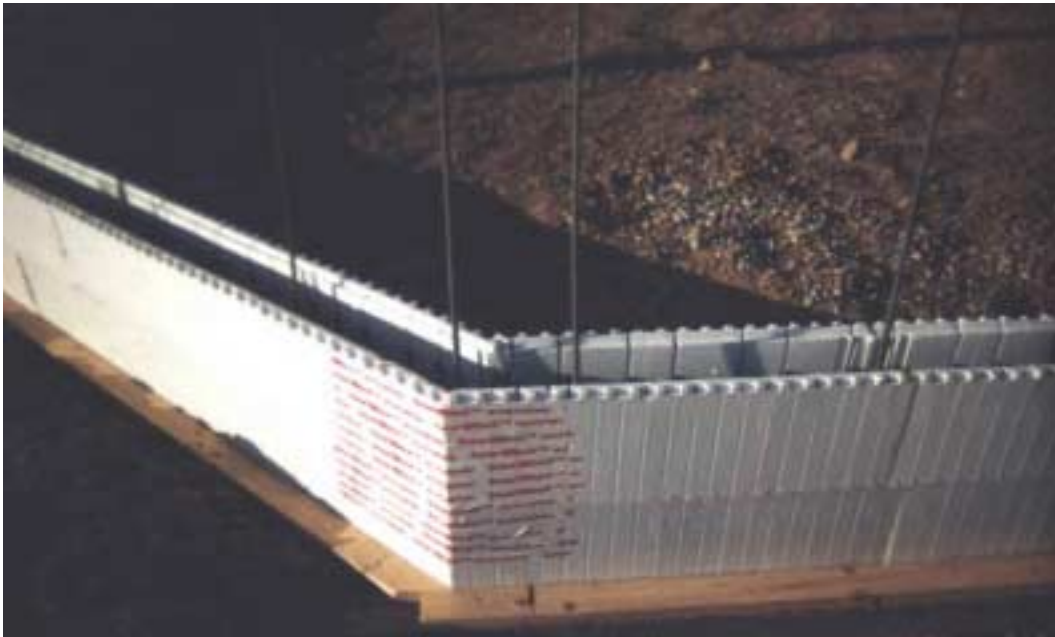
Angles or curves are easy with SmartBlock.
