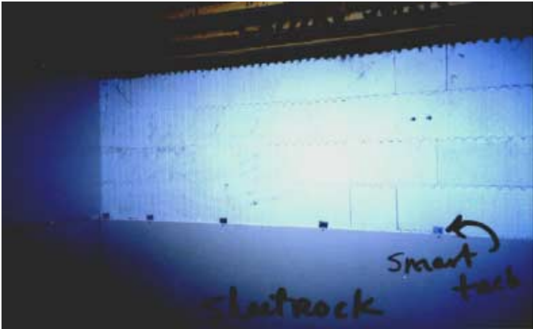
Attach drywall to our SmartTach or plastic connectors.
