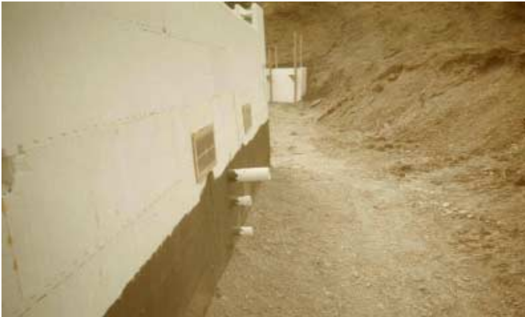
Service penetrations should be in prior to the pour.
