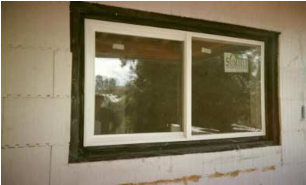
Flash windows with a membrane just as usual.
