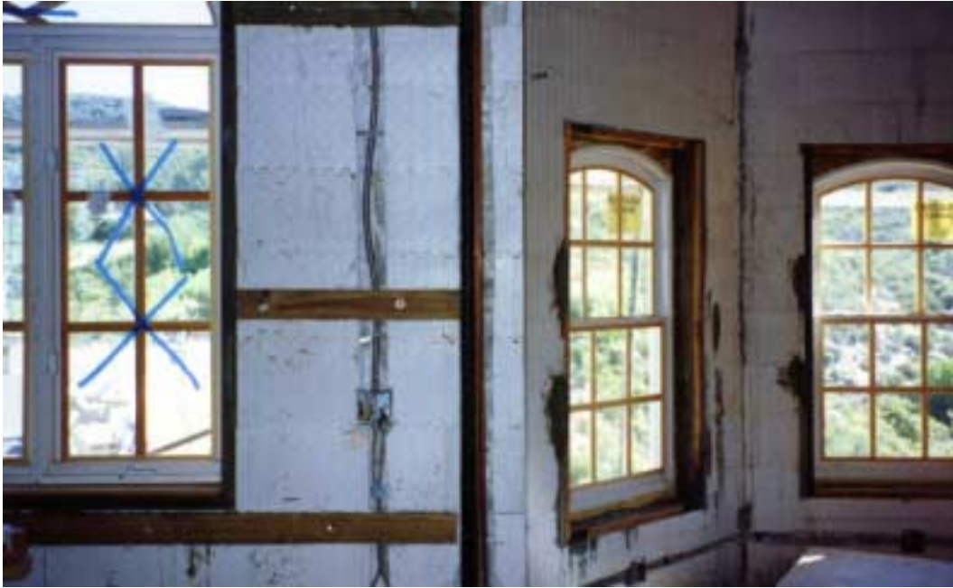
Route out foam for electrical and plumbing chases.
