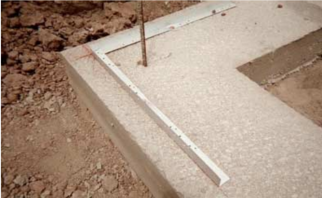
Level footers start with a chalk line and cleat.
