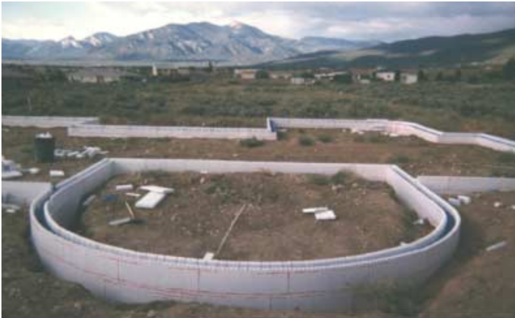
Interior cuts create curves and insulated slabs.
