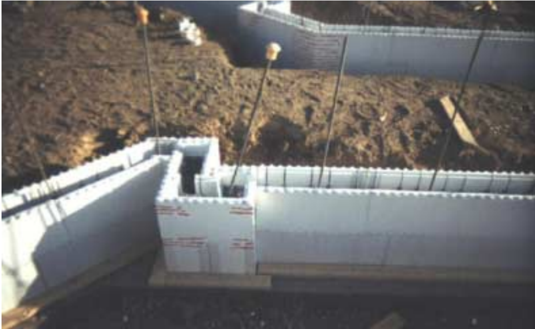
SmartBlock is fast and easy when forming complex designs.
