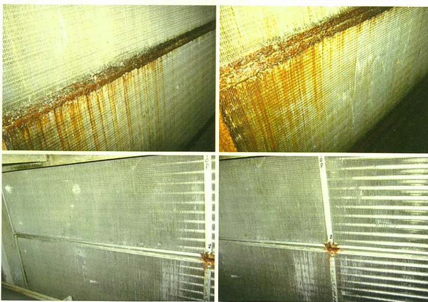
Figure 9: Professional deep coil cleaning restores 6 row coils to original condition
