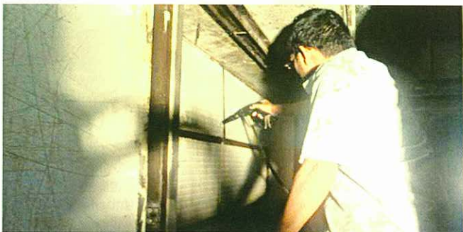
Figure 6: AHU cleaning of 6 row coil with a small gun
