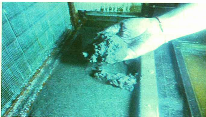
Figure 10: Mold cleaning in the tray after deep coil cleaning
