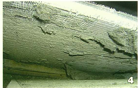
A condenser coil in need of cleaning
