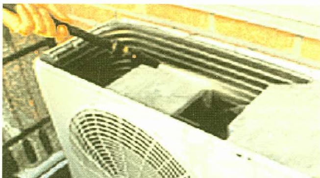
Figure 5: Cleaning in a tight space with low pressure and low water flow
