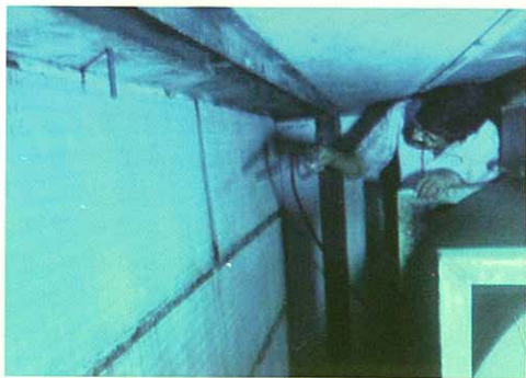
Figure 7: AHU coil cleaning at back side
