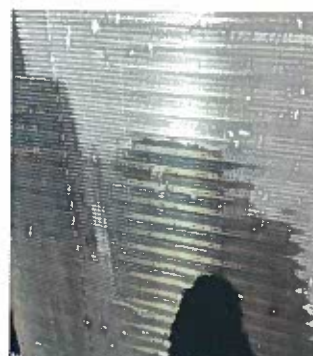
Figure 14: Restored coil after fin cleaning and nano coating
