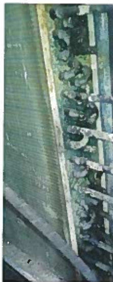
Figure 11: Old header with paint and rust oxides
