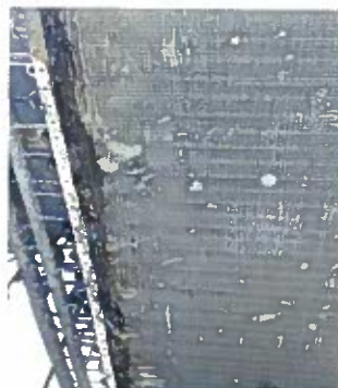
Figure 13: Old coil with dirt and corrosion
