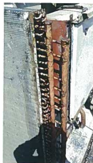
Figure 12: Chemically cleaned and coated header
