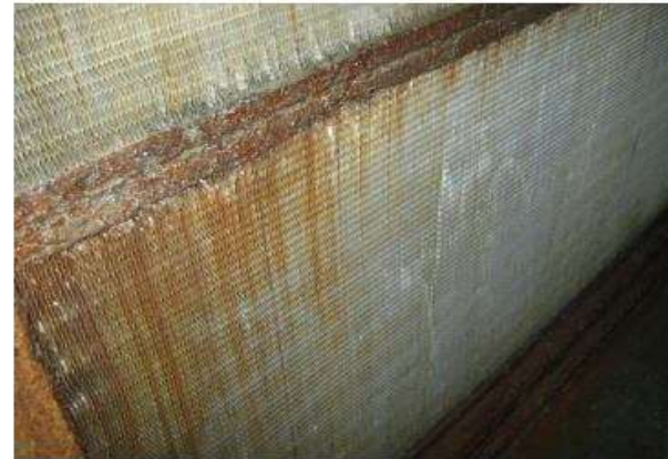
Tube visibility after cleaning is 3 row deep
