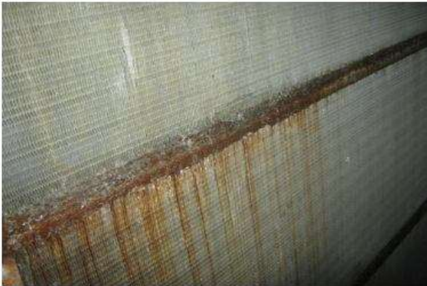
Cooling coil Snaps after cleaning
