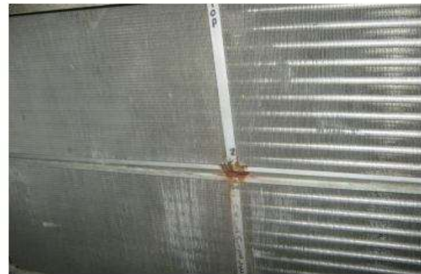
Tube visibility after cleaning is 3 row deep
