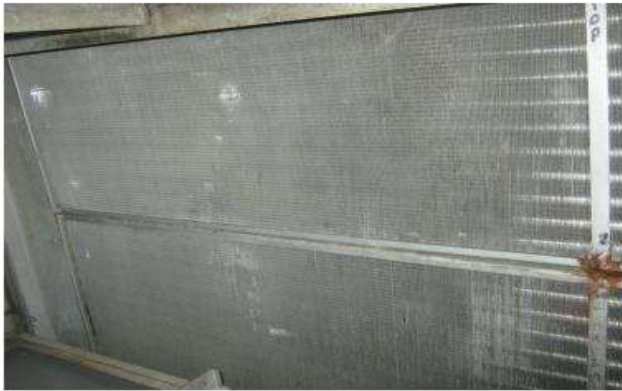
Cooling coil Snaps after cleaning
