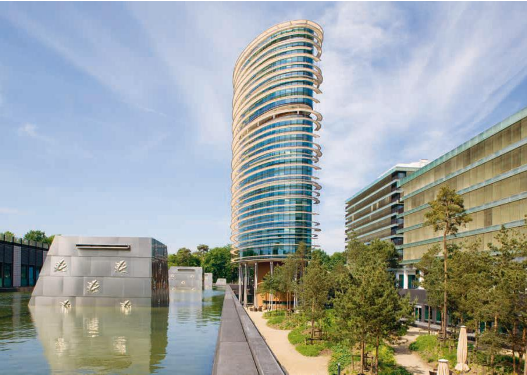
EPDM waterdak Walterbos-complex, Apeldoorn.
