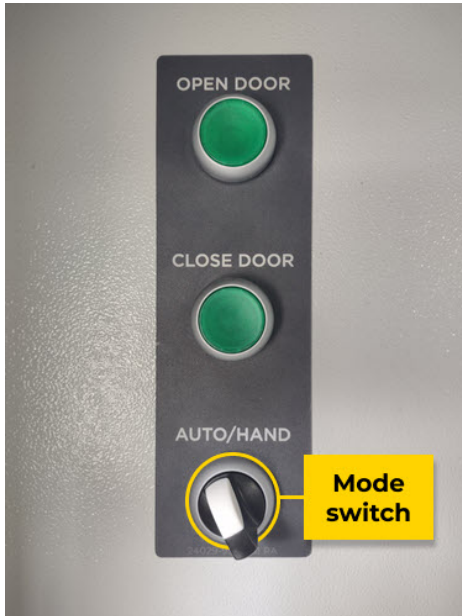
Spot door operating controls on the Industrial Control Panel.
