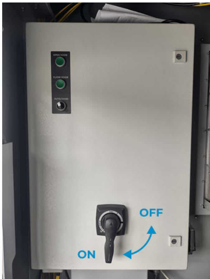
Power switch for the Spot Station.
