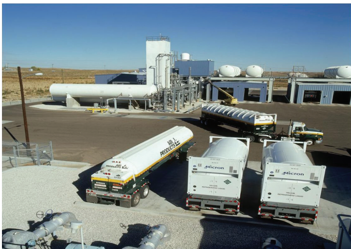
FIGURE 2.3 U.S. liquid helium plant (in the rear), helium tankers (attached to the truck and on the left), and International Organization for Standardization (ISO) containers for overseas shipment (middle and right). SOURCE: Air Products and Chemicals, Inc.
