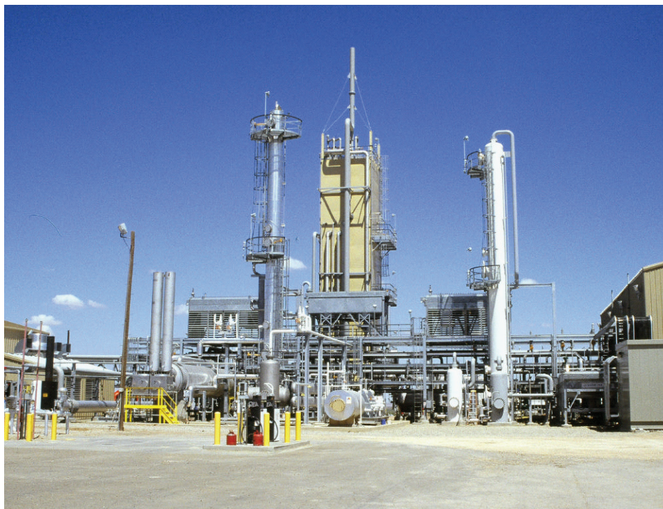
FIGURE 5.2. Crude helium enrichment unit installed to provide a more reliable flow of crude helium to refineries. SOURCE: U.S. Department of the Interior's BLM.
