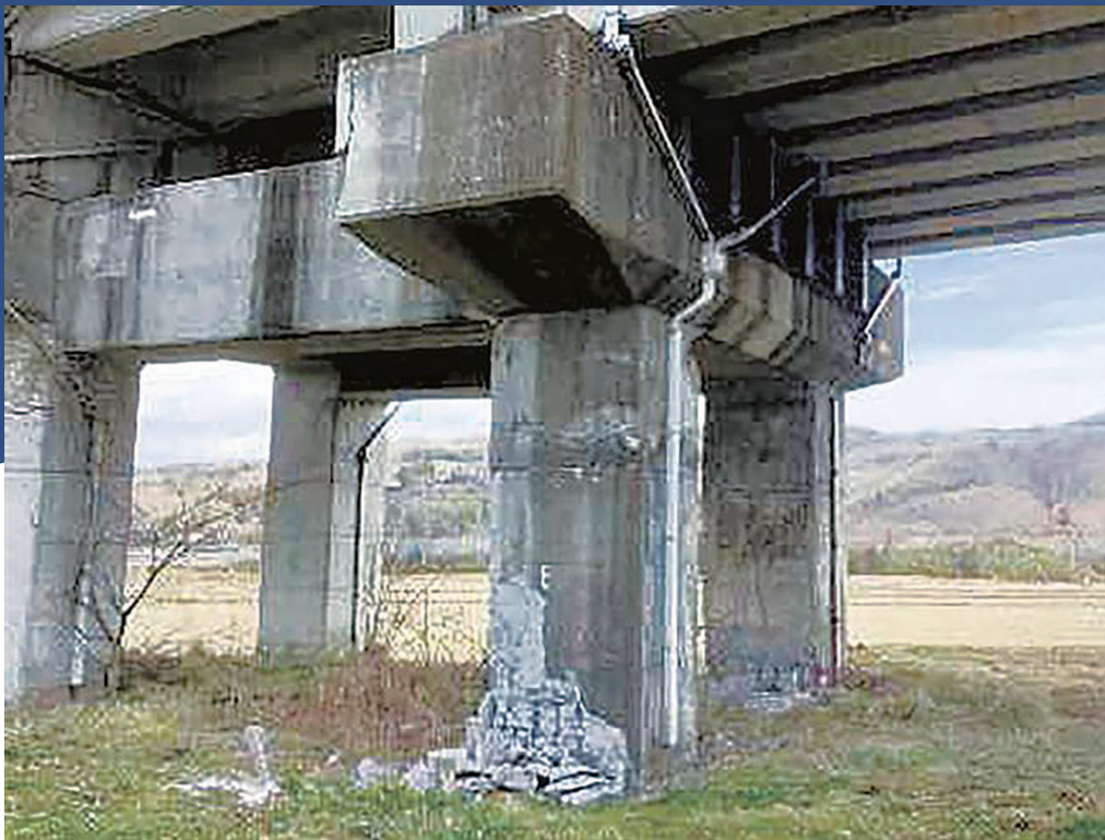
Rupture and rust juice due to rusting of steel frame , Hydrolysis of paint with cement alkali, large amount of efflorescence, etc
