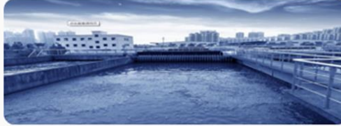
SEWAGE TREATMENT TANK
