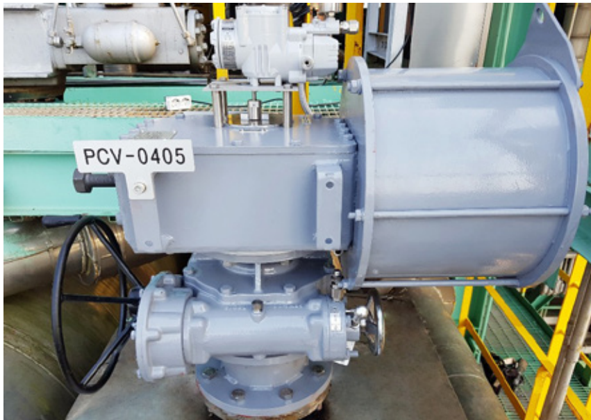
Declutchable Worm Gear Manual Override
