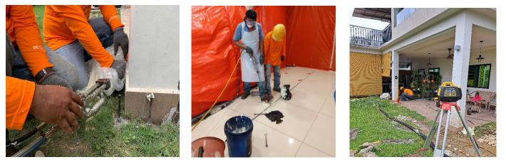
Rotary laser level is a precision instrument used to establish a consistent horizontal or vertical plane across a site. During PU injection, it helps monitor and control the level difference of the structure by emitting a 360-degree laser beam. A level indicator receiver is placed on the structure to detect this laser beam, providing real-time feedback on any movement or lifting as the PU foam is injected.
