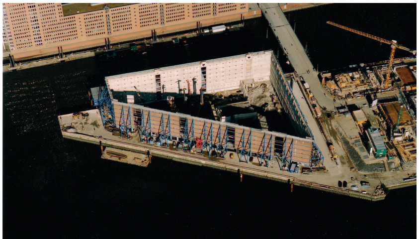
fig 27. Aerial photo of demolition process
