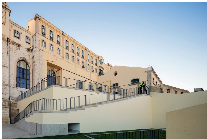
fig 10. Facade view, Chiado Lisbon
