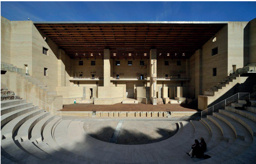
fig 14. Aereal view of Sgunto theater
