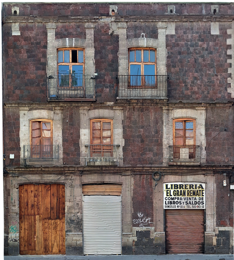
fig 44. Photogrammetry of the facade of Donceles 81
