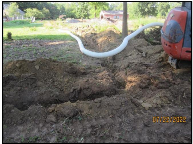
*The main line going down to the road ditch. Five lateral lines come in from each side.*
