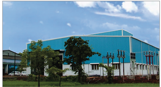
KOLHAPUR - MAHARASHTRA PIPES
