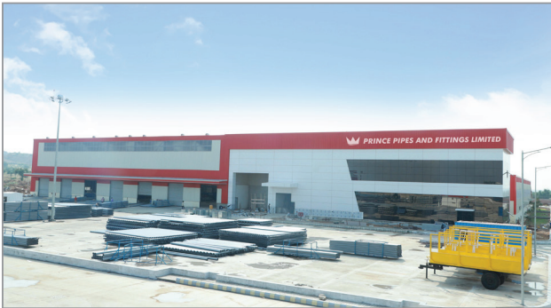
JOBNER - RAJASTHAN PIPES & WATER TANKS
