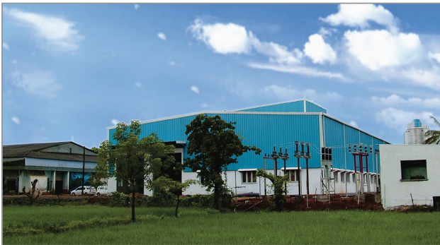
CHENNAI - TAMIL NADU PIPES
