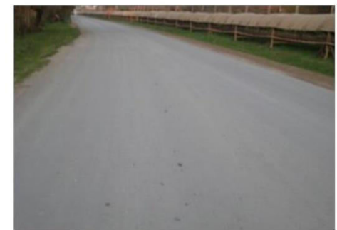
Road covered for longer life
