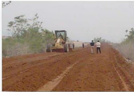
Scarification of the soil
