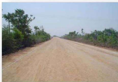
Compacted road (ready to be used or set for any type of topping)
