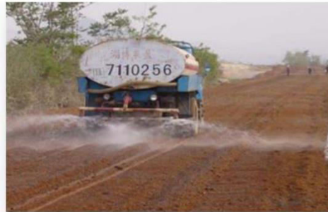
Applying the mixture
