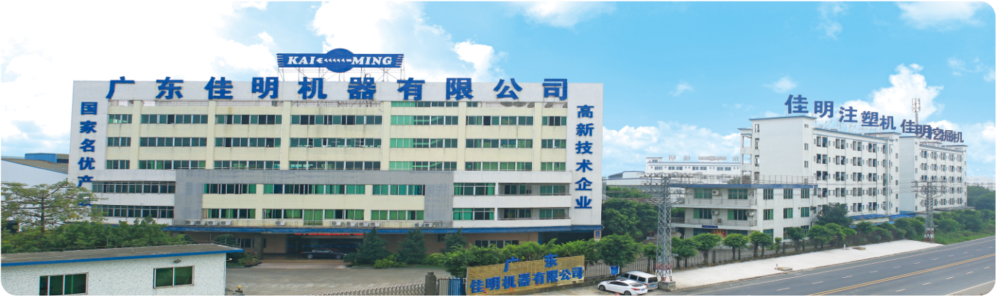
佳明一厂 KAIMING PLANT 1
