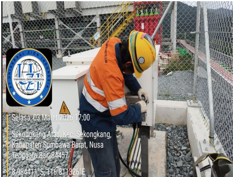
Electrician Power Cable / Lokasi 3100
