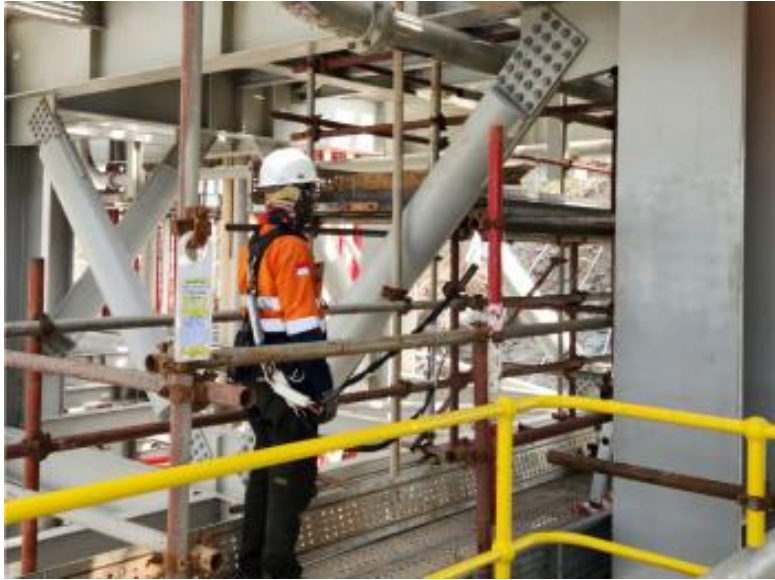
Performing internal inspection of scaffolding structures. / Lokasi 3100
