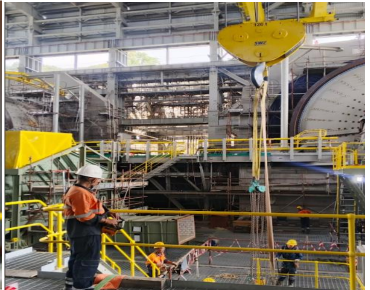
Carrying out material lifting operations using an overhead crane. / Lokasi 3100
