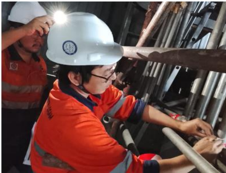
Conducting an inspection of fine holes that are not coated with paint./ Lokasi 3600 Painting Inspector
