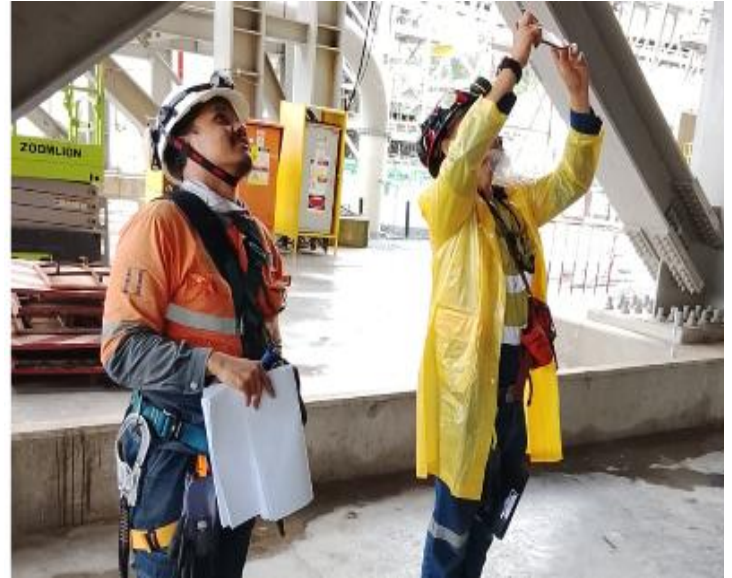
Conducting pipe inspection together with the client./Lokasi 3300
