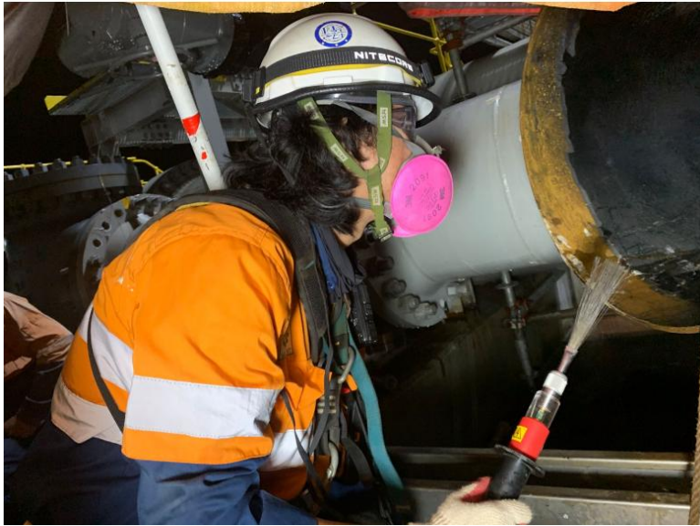
Conducting an inspection of fine holes that are not coated with paint./ Lokasi 3600 Painting Inspector
