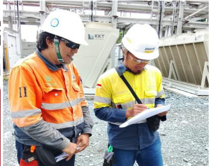
Conducting pipe inspection together with the client./ Lokasi 3300
