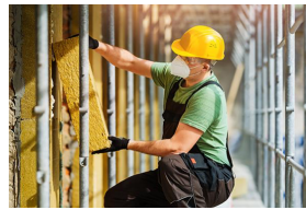
Renovation of public buildings
