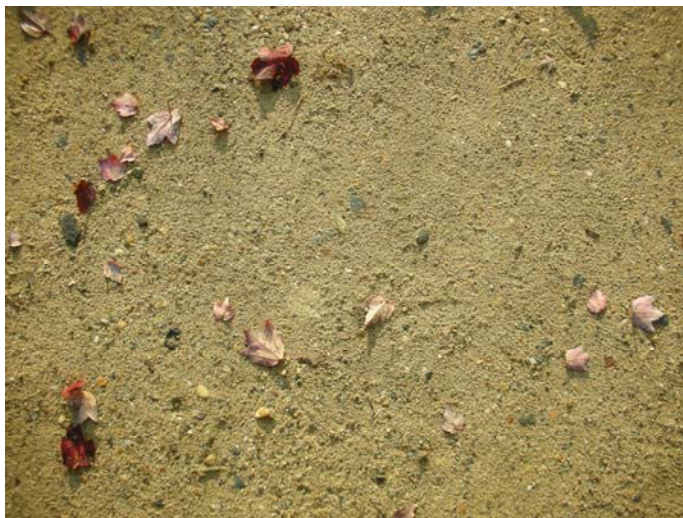
Figure 3. View of the sand like surface. The path is compacted stone dust and does not show bike tracks or foot prints. Minute Man National Park (Concord).
