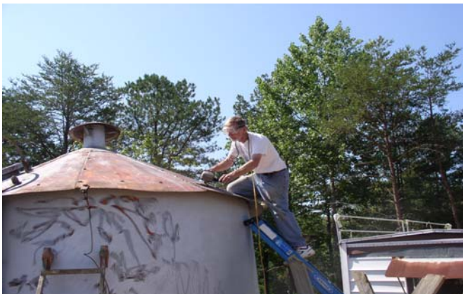
Bill Hawkins working on the water tank
