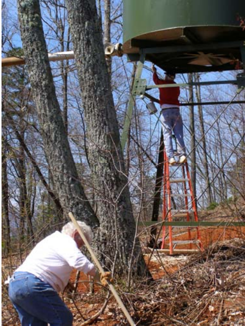
Ron & Linda Tadlock working at the water tank
