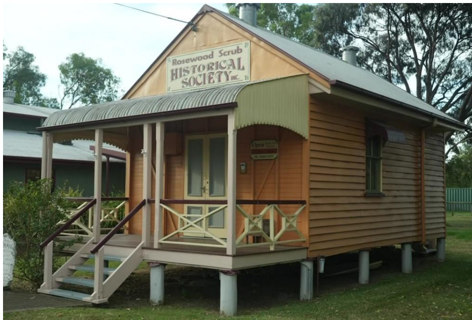
The Rosewood Scrub Historical Society Building was built in 1913 in Marburg, Ipswich. (ABC News: Charlie McLean)
