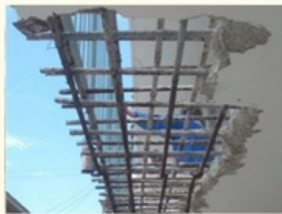
Concrete Spalling Repair
