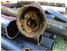
Cast Iron Repiping
