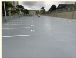
Painting and Waterproofing
