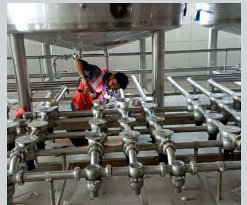
Valve Battery Skid
