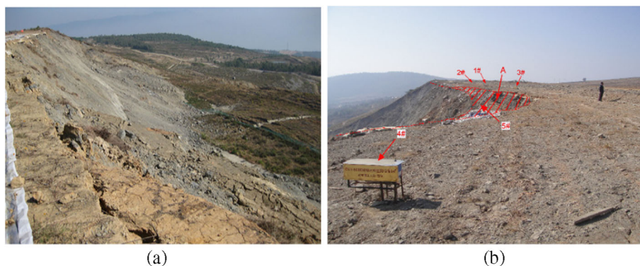
Fig. 25 a Field photo showing a 15-cm-wide crack at the trailing edge of the landslide. b Scene photo of one collapsed body
