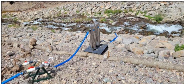
Figure 5. Water flows through the manifold through bag filters and into the stream
