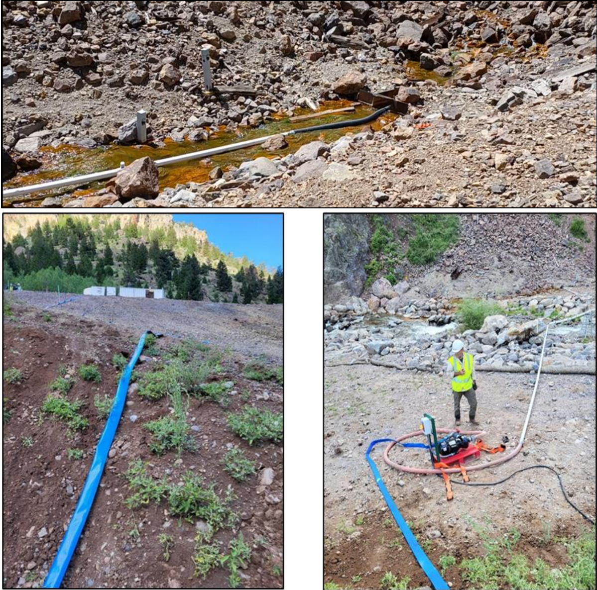
Figure 2. Water conveyance system from flume to lift pump and uphill to treatment
