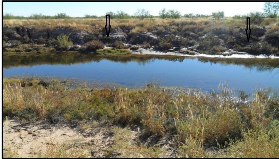
Looking at eastern side of later cattle crossing broken down embankment
