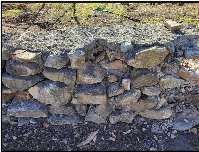
Re-purposed Building Stones For Dam
