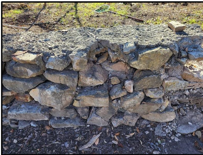
Re-purposed Building Stones For Dam
