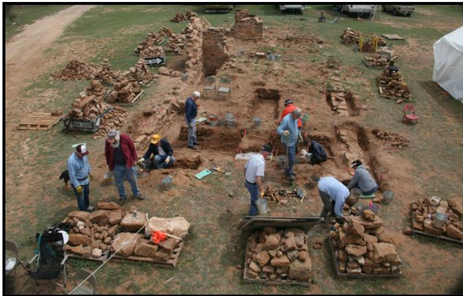
Walls removed and ground excavation commencing
