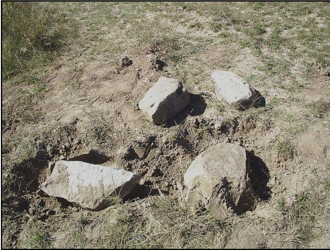
Unearthed limestone was probably used for footings of pier and beam construction
