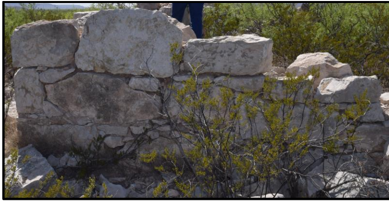
Fully Cut Blocks on Base of Wall
