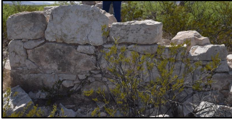
Fully Cut Blocks on Base of Wall
