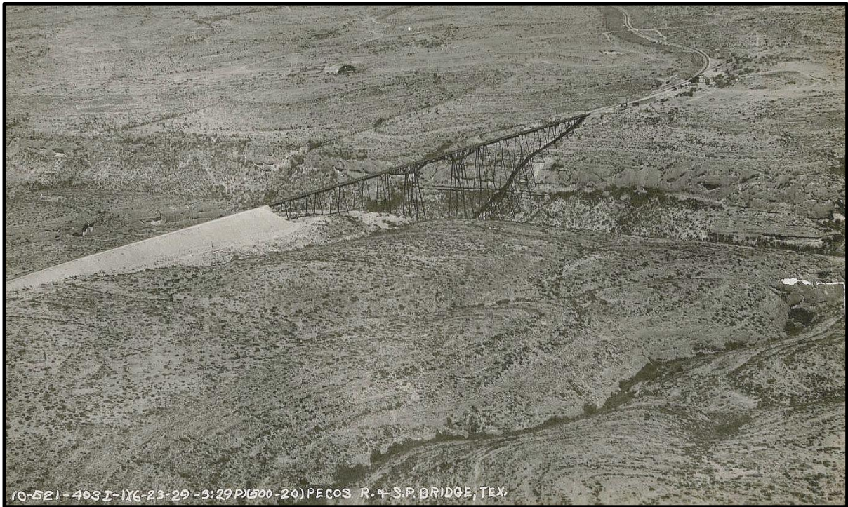
1929 Army Air Corps Photo of Pecos River Railroad High Bridge (1922 depot in upper right of photo)
