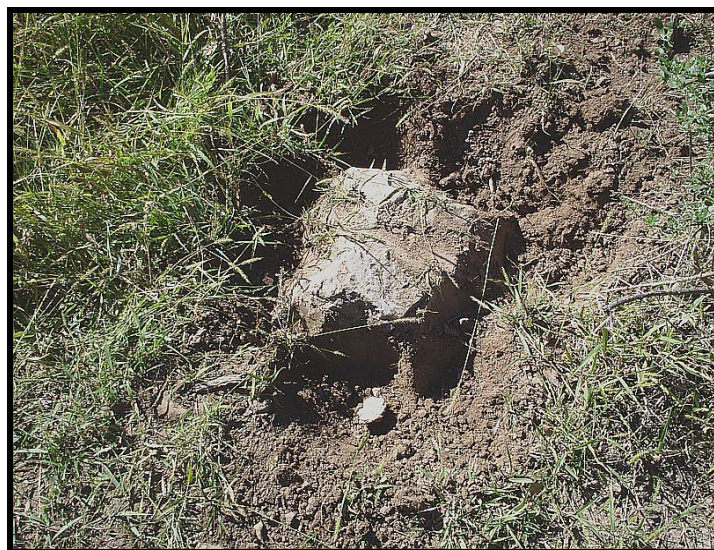
Figure 21: Unearthed cornerstone used for footing of pier and beam construction
