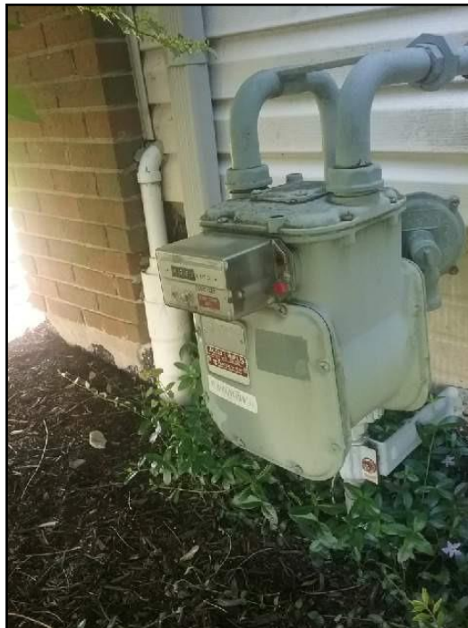
14. Gas supply and emergency shut off
