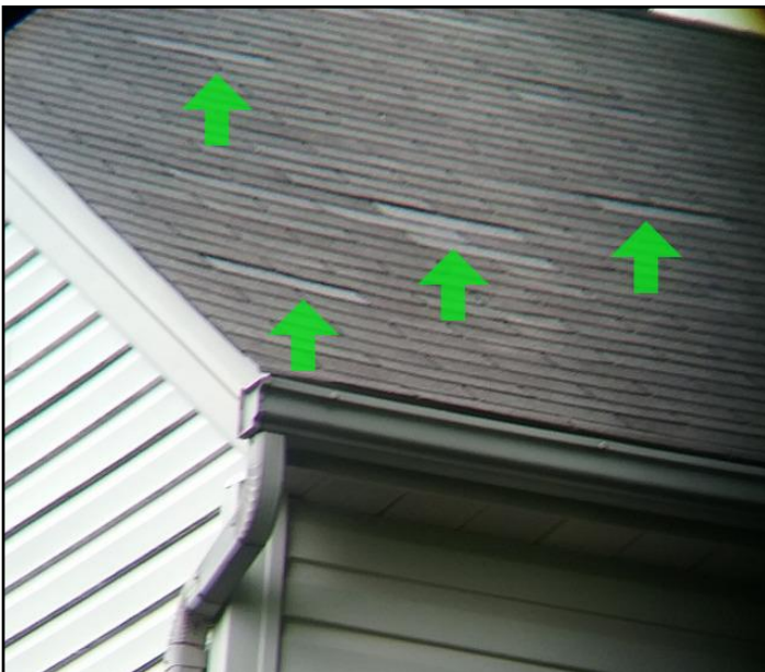
1. missing shingles: NW roof
