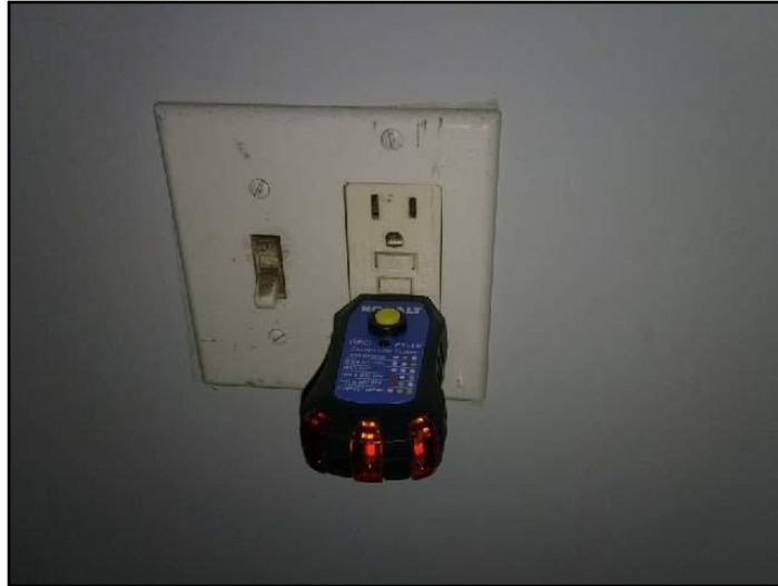
11. GFCI in garage operable
