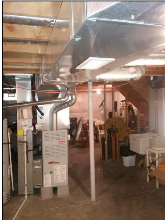
12. Forced warm-air heating with extended plenum
