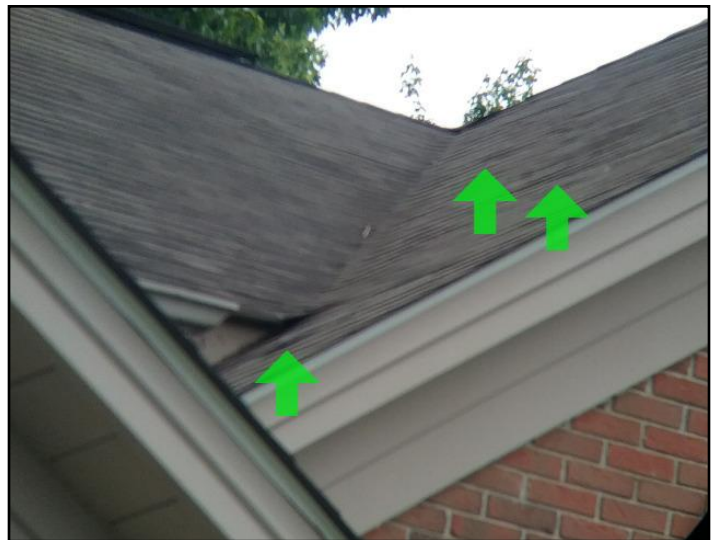
2. missing shingles: SE roof
