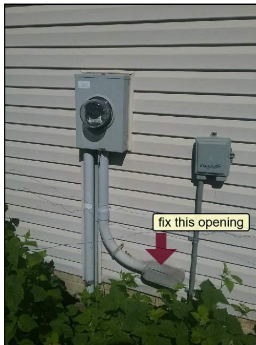
10. damaged hardware at service entrance
