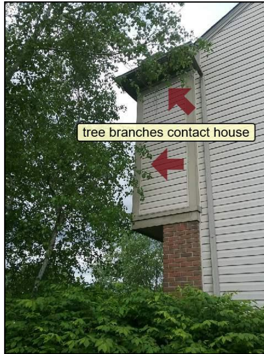
7. birch tree contacts house and gutter
