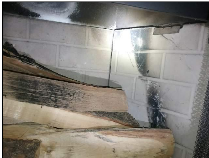
17. fire-brick lines firebox
