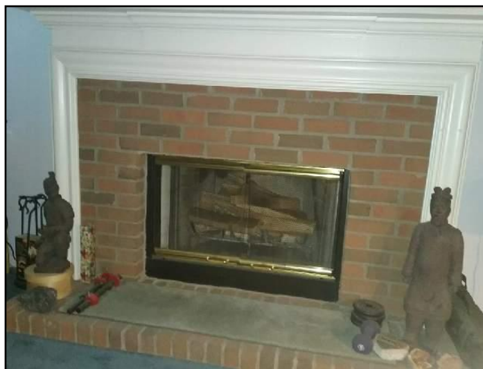
21. masonry fireplace with carpet on hearth
