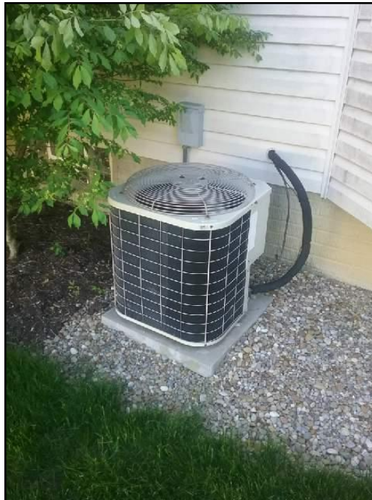
22. compressor / condensor unit
