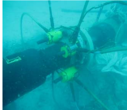
Subsea Bolt Tensioning
