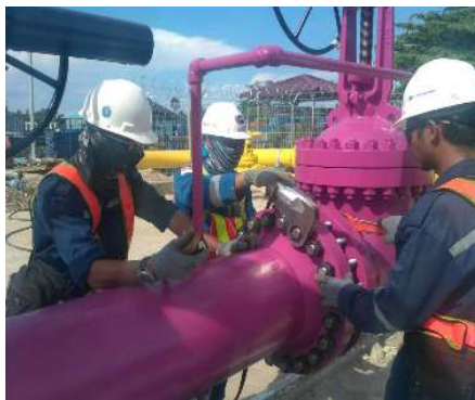
Hydraulic Torque Wrench
