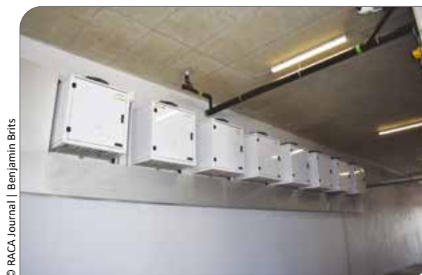
Cold and freezer room condensers.
