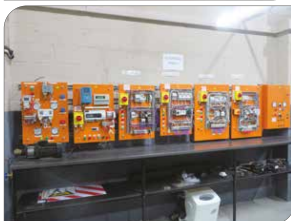
Training is given on different electrical panel layouts.
