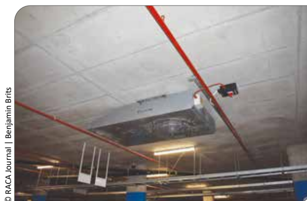
A jet movement fan in the underground parking area.
