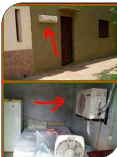
Supplied by DQT Air / W Air & Refrigeration
