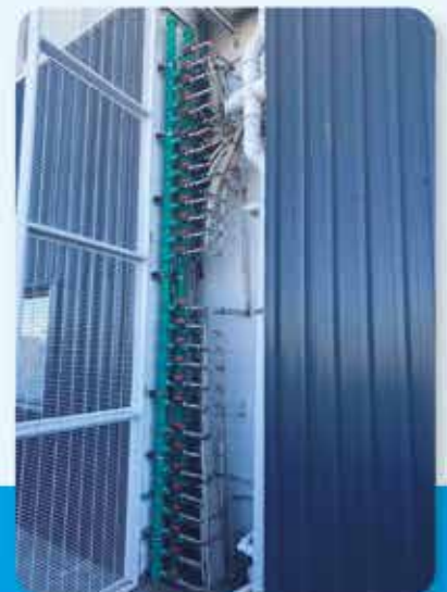
All Photos of the installation at the site.
