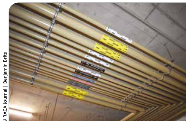
Medical gas pipe reticulation.
