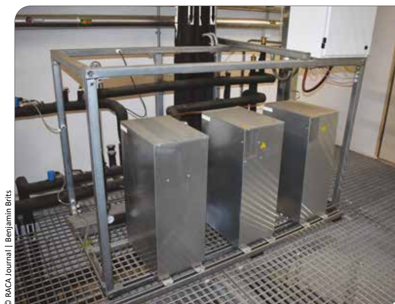
One of the VRF booster and HEX unit installations.
