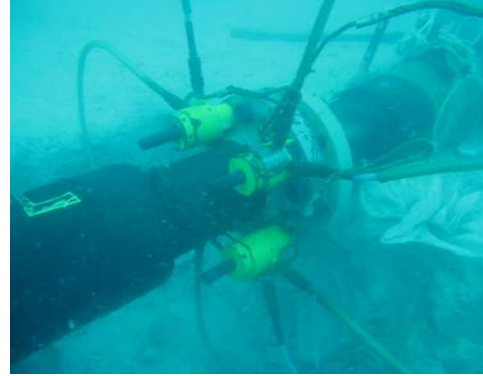
Subsea Bolt Tensioning
