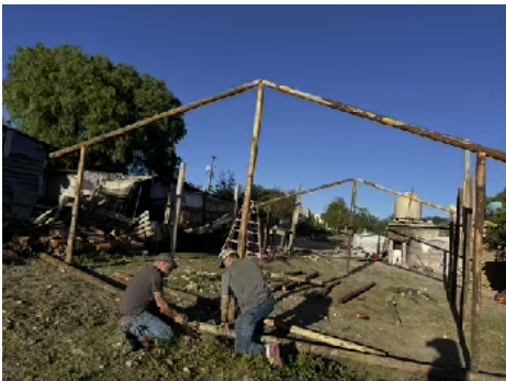
Building church in La Presa
