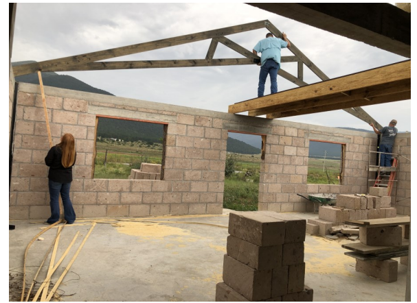
The Browns helping with the rafters (scissor trusses)
