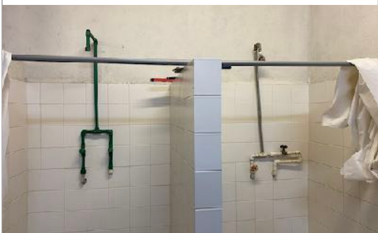
New plumbing vs old plumbing in the camp dorm
