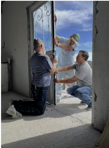
New church door in Puerto Mexico
