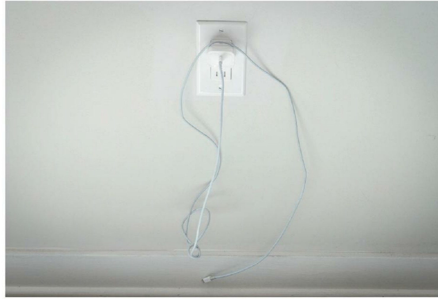
A phone charger plugged in a Center City apartment. In Fairmount, Janice Simonsen said she is making sure she unplugs everything after receiving a more than $300 electric bill for a 750-square-foot unit. Jessica Griffin / Staff Photographer
