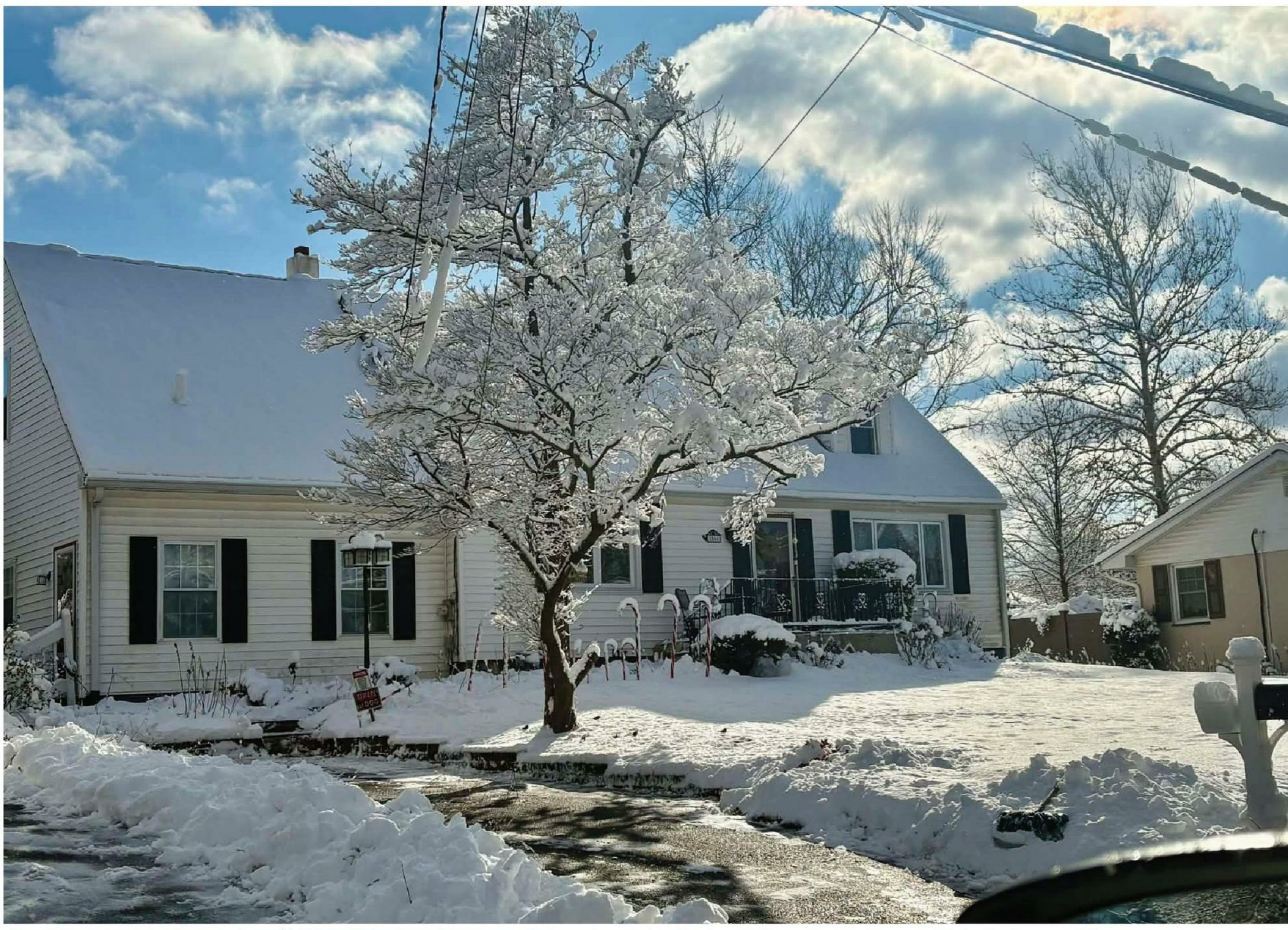
Carol Capriotti paid more than $700 in February for gas and electric service for her Willow Grove home, which she heats with a gas-powered boiler. Courtesy Carol Capriotti
