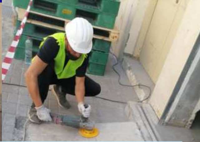
Concrete ramp repair work Safco warehouse DIP
