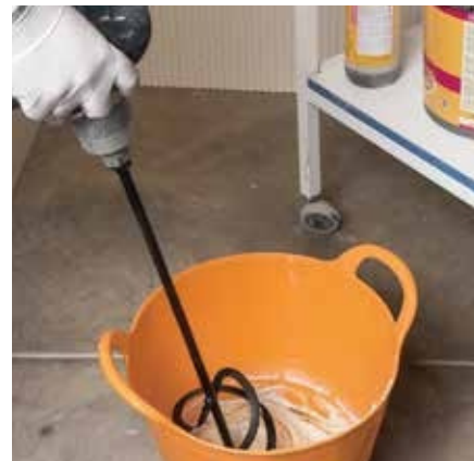
2. Mix the hardener and polyurethane adhesive thoroughly at a ratio of 10/1.
