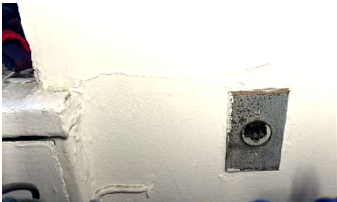
15 amp 125 volt ancient outlet for window a/c
