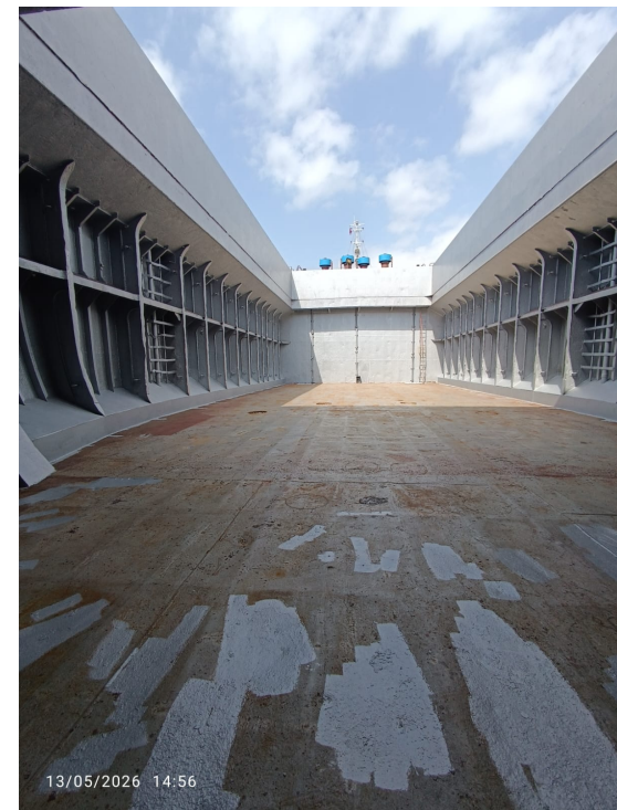
BACKSIDE OF HOLD NO.1
