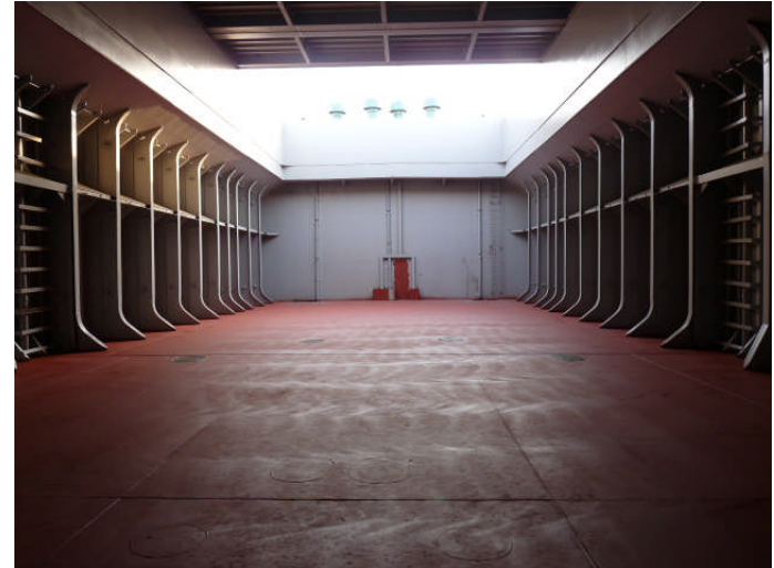
BACKSIDE OF HOLD NO.1 (hatch cover was not totally opened when taking pictures)
