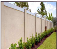
Compound Wall for Entire Layout
