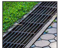
Open Drainage System
