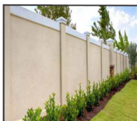
Compound Wall for Entire Layout
